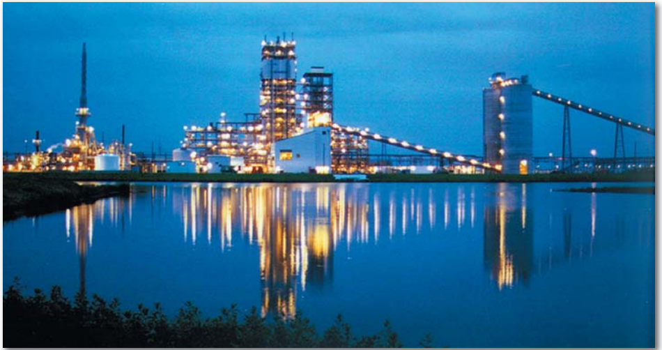
Tampa Electric's Polk Power Station
